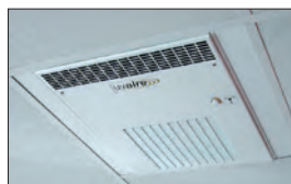
Drop ceiling installation
